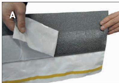
**POSA DI ISOLMANT FASCIA PERIMETRALE TECNICA DOPPIO SPESSORE SU SOLAIO.**
